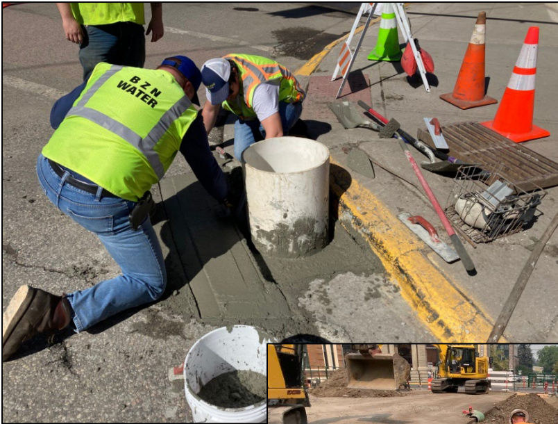
Graphic 2.0.1: Stormwater Inlet Retrofit
