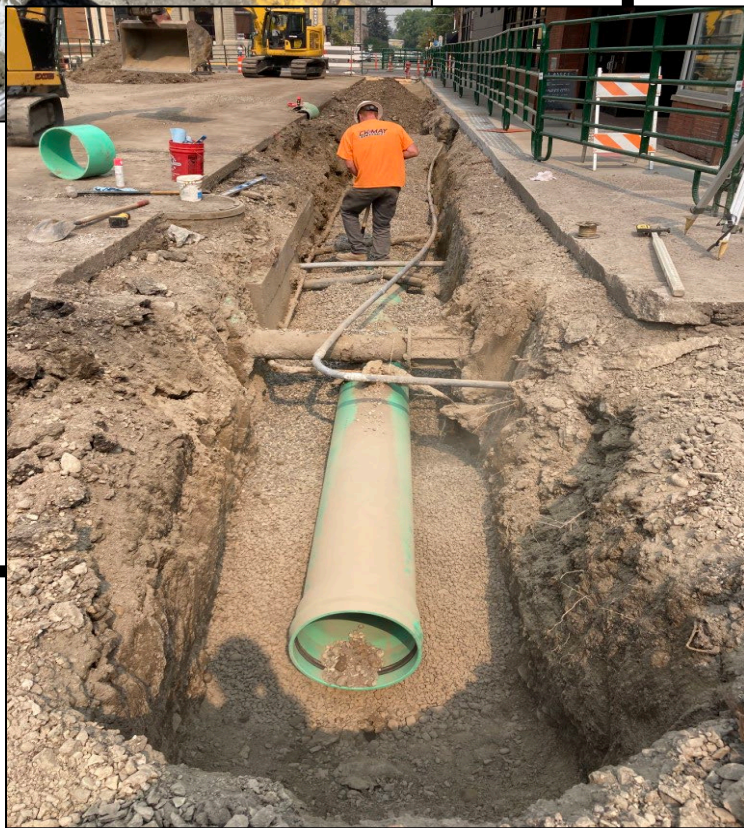
Graphic 2.0.2: South Tracy Ave. Storm Sewer Pipe Replacement
