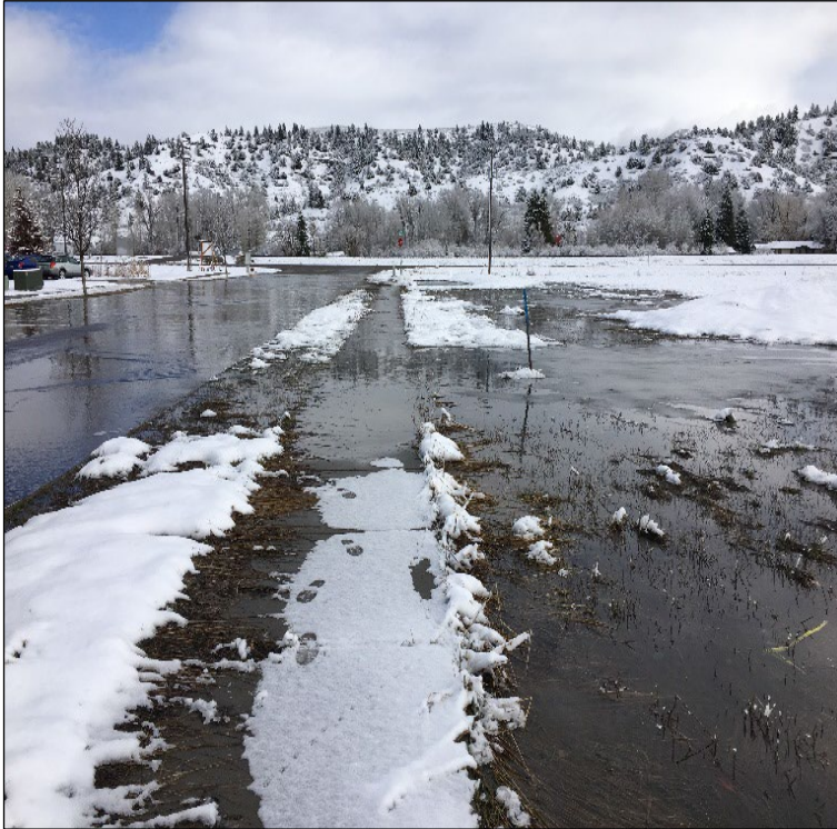
Graphic 1.0.1: Street flooding resulting from clogged infrastructure
