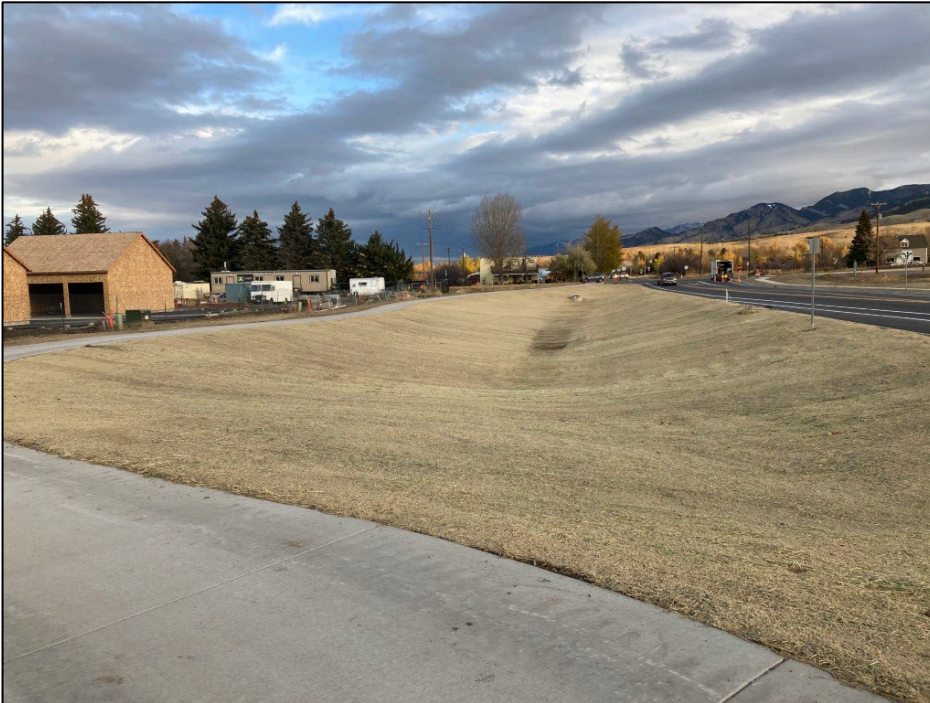
Graphic 5.0.1: Recently constructed and stabilized stormwater pond
