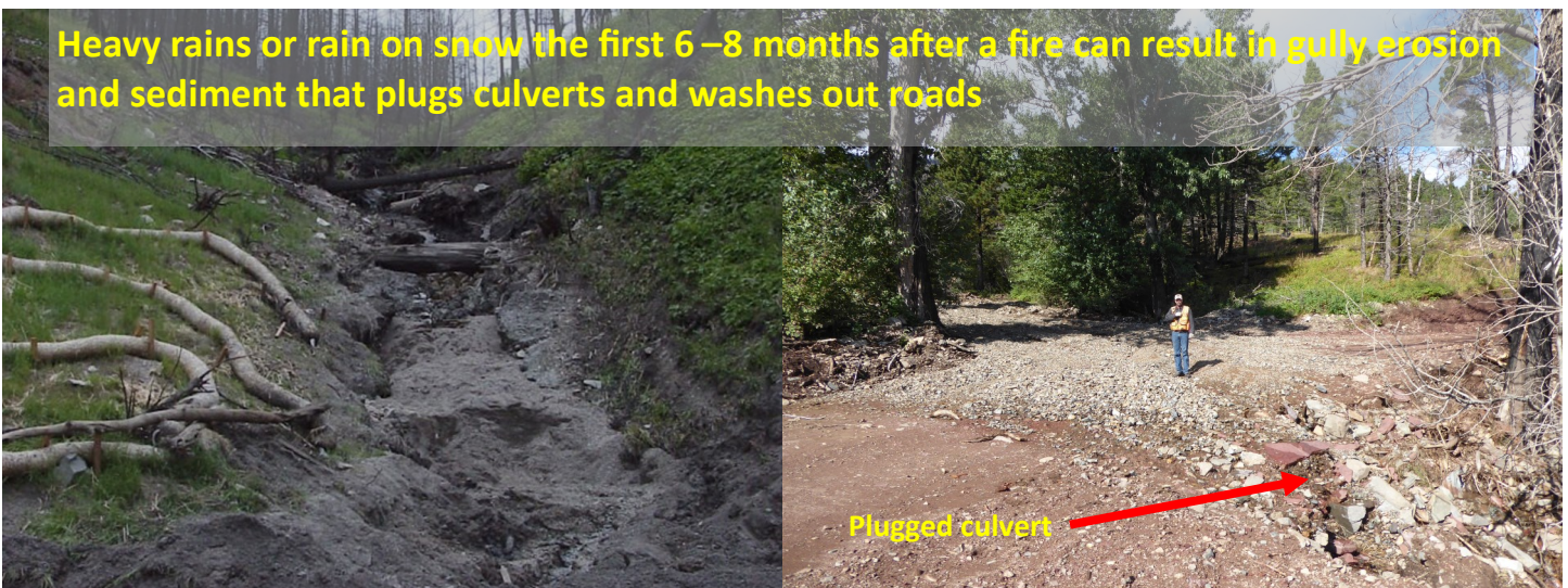
Picture 16. Increasing soil water absorption and decreasing surface water flow in the upper reaches of a drainage is critical to reducing fire related flood events. Accumulated water can break through lower drainage erosion barriers.
