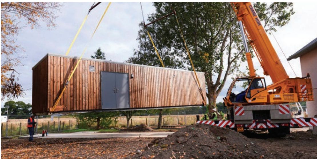
FIGURE 5: Installation of a containerized system
