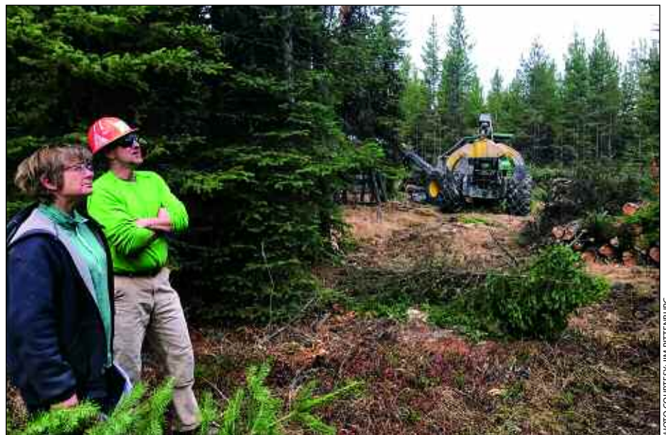
Lorna Rittenburg and Mark Boardman, working with the crew from Stoltze Lumber company, lay out the skid roads that will later become recreational trails.
