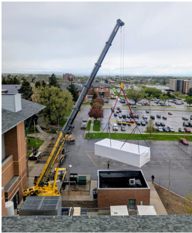
A giant crane lifts the “Fish Pod” over Chem Stores
