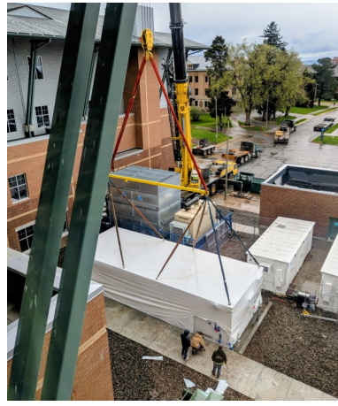
The “Fish Pod” is carefully lowered on to its foundation.
