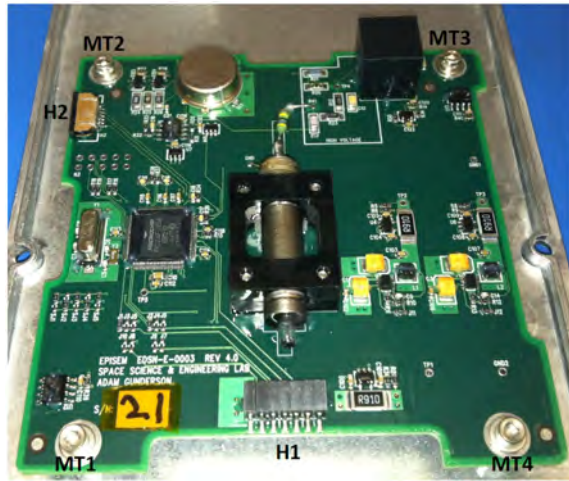
Figure 30: Test points measured to ground in the power and unpowered portions of the Safe-to-Mate test.
